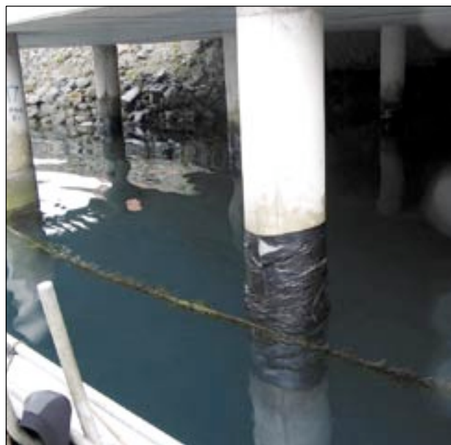
Containment: Pile wrapping as an incursion response tool.
